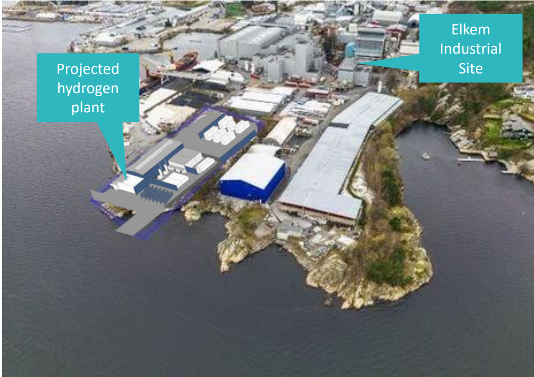
Located on Elkem's industrial site in Kristiansand
